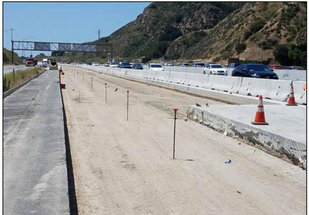
**These lanes in the Newhall Pass are shown after being fully excavated in preparation for the new pavement. Photo courtesy of Caltrans**
